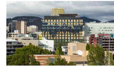
Royal Hobart Hospital Redevelopment, LYONS WITH TERROIR
