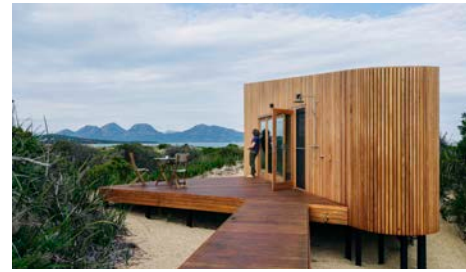
Dolphin Sands Studio, MATT WILLIAMS ARCHITECTS
