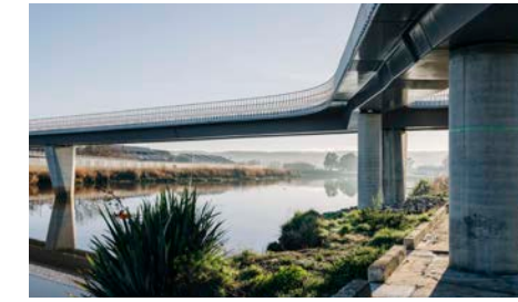
North Esk Pedestrian Bridge UTAS, JOHN WARDLE ARCHITECTS
